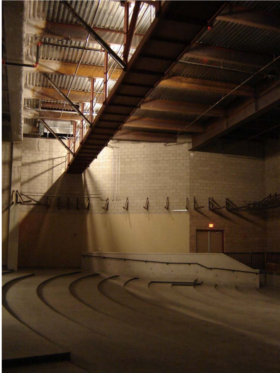
Golden Valley High School Theater – Prior to Construction
