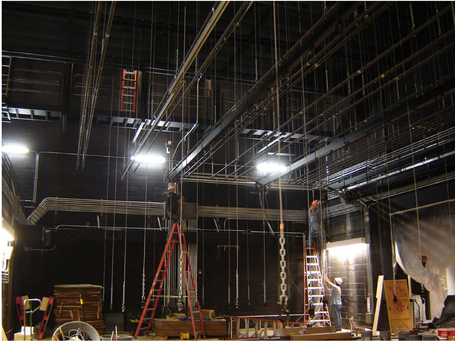
Golden Valley High School Theater – Stage Rigging Installation Underway
