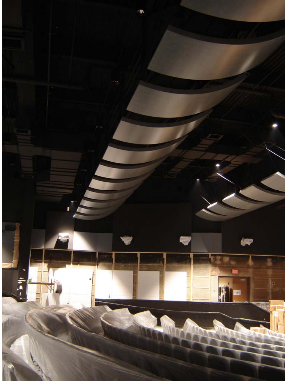
Golden Valley High School Theater – During Construction
