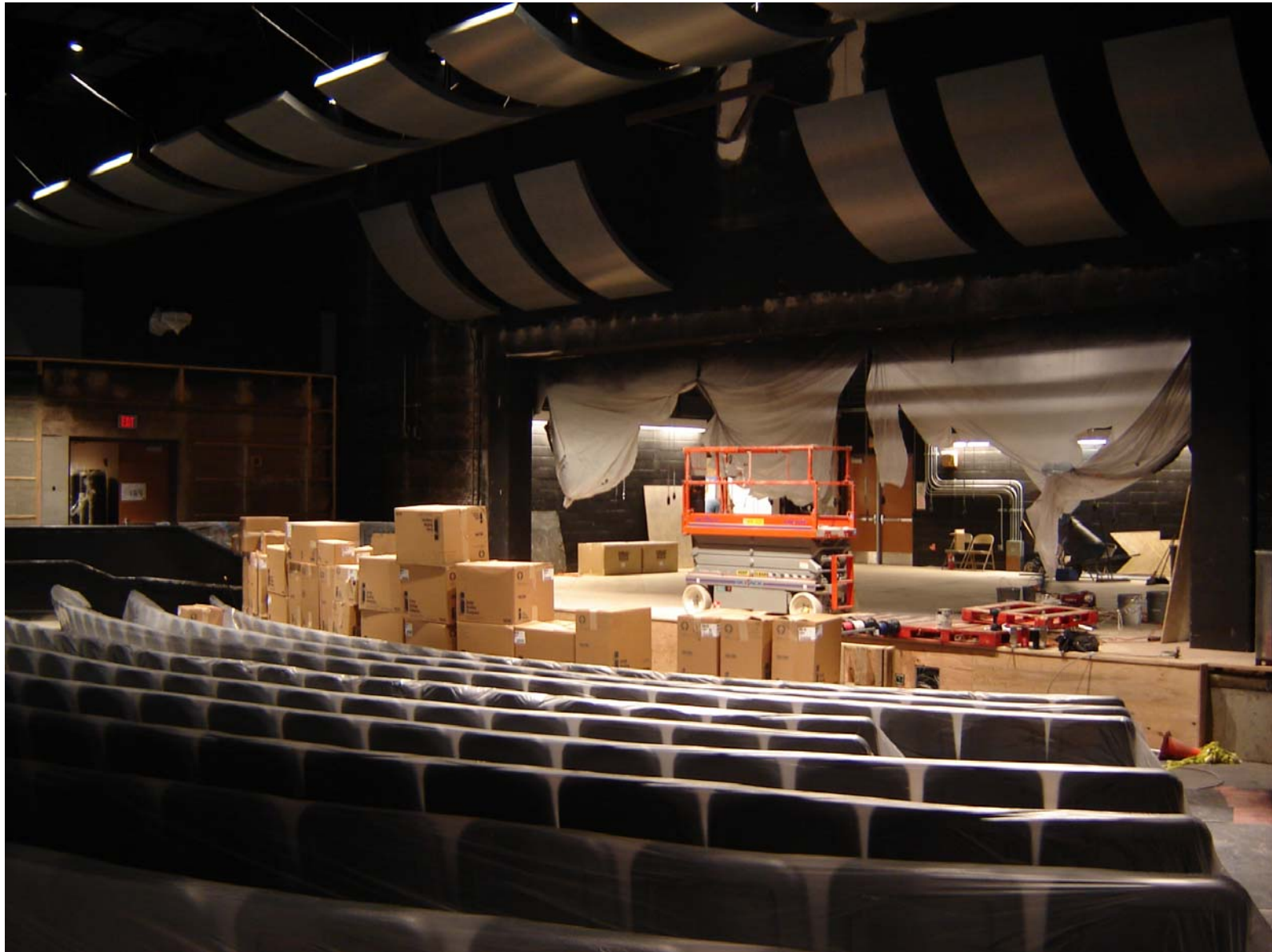
Golden Valley High School Theater – Seating Installation Underway
