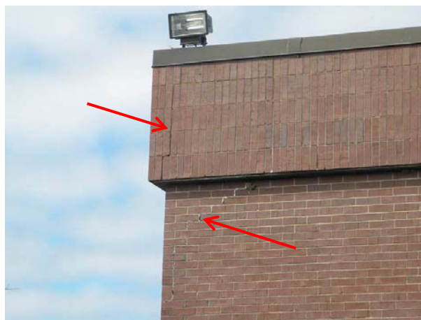
Figure I-02: Cracked joints and split brick at outside corner.
