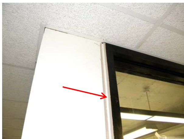
Figure H-23: Joint at steel frame to concrete. (Note stripes of gray epoxy encapsulant at either side of existing joint applied in 2011.)
