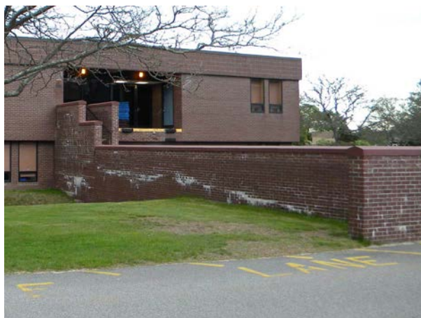
Figure I-08: Efflorescence at exterior brick walls to loading dock.
