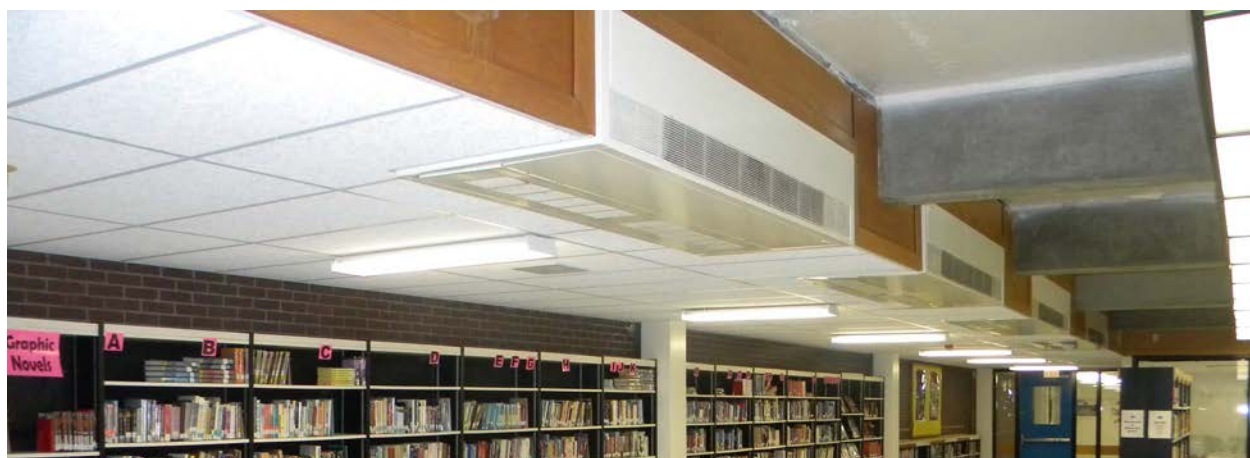
Figure H-34: Acoustical tile ceiling and plywood fascia at Media Center.
