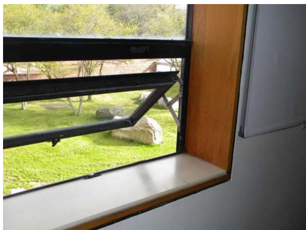
Figure G-08: Interior wood trim and Corian stools at typical Type 'A/A1' windows.
