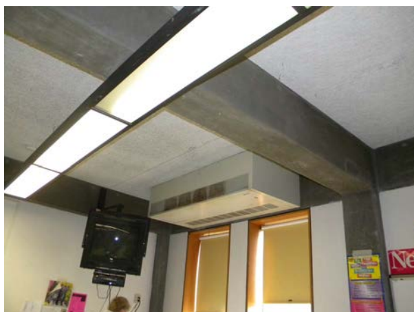
Figure C-12: Original Tectum form plank ceiling at typical classroom.
