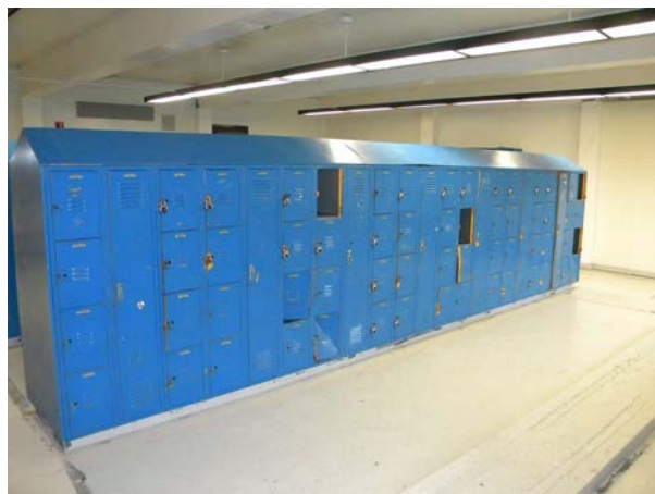
Figure I-05: Damaged original boys' locker room lockers, also repainted.
