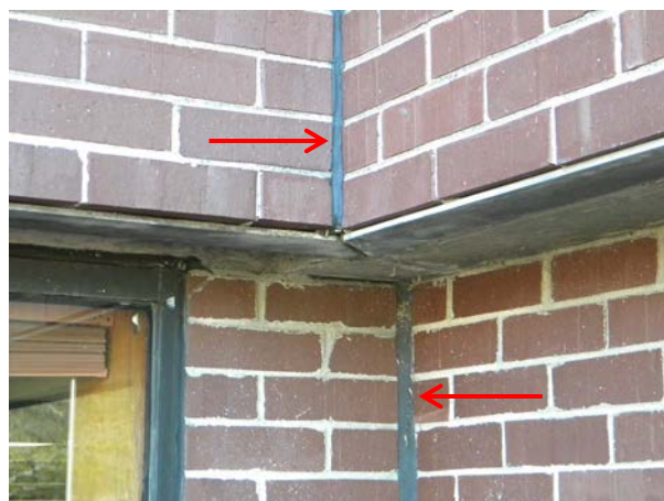
Figure C-09: Caulk at exterior expansion joints removed and replaced.
