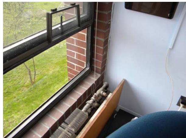
Figure H-27: Finned tube radiator and plywood cover at typical Type 'B' windows.
