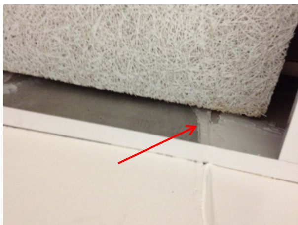
Figure G-38: EnviroScience reported that care was taken to remove foam fillers above existing suspended ceilings.
