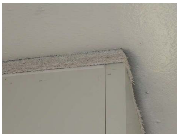
Figure C-22: Enlarged view of Tectum form plank above unit ventilators.
