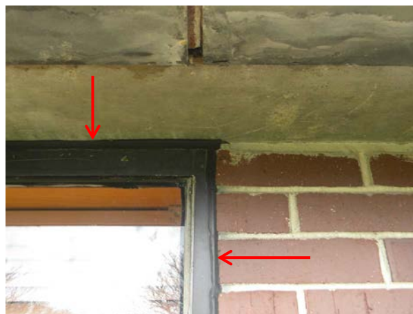
Figure C-03: Exterior perimeter caulk at typical windows removed and replaced.
