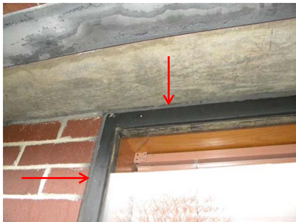
Figure C-01: Exterior perimeter caulk at typical windows.
