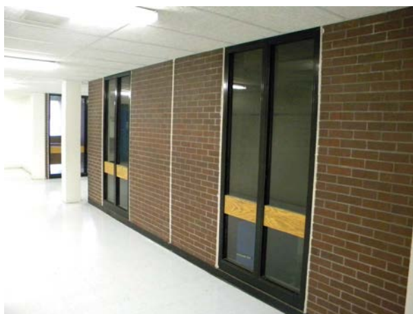
Figure D-03: Interior brick adjacent to expansion / control joints and fixed lite frames.
