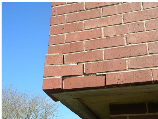
Figure I-01: Displaced brick veneer at outside corner.
