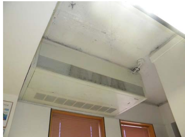
Figure G-23: Typical classroom unit ventilator with Tectum form plank above.
