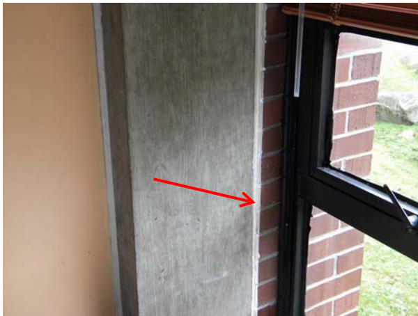
Figure H-19: Joint at brick to concrete at piers.
