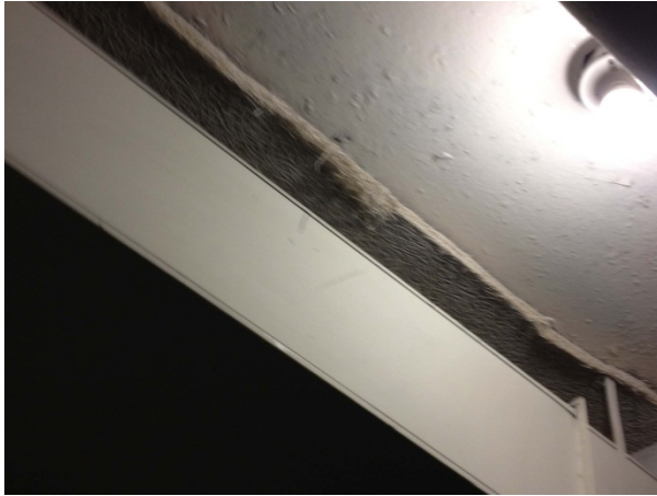
Figure G-24: Tectum form plank above mechanical equipment and ductwork in Gymnasium Storage Room 141.
