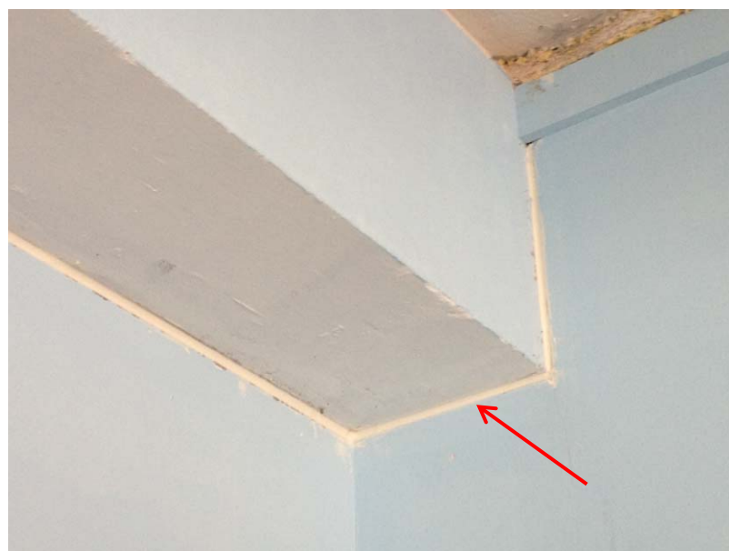
Figure C-29: Original foam filler removed at joints between concrete structure and plaster partitions. Joints cleaned out, encapsulated, and resealed with new caulk.
