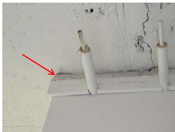
Figure G-20: Approximately 2" thickness of Tectum form plank remaining at top of typical partitions following the 2011 PCB Source Removal Project.
