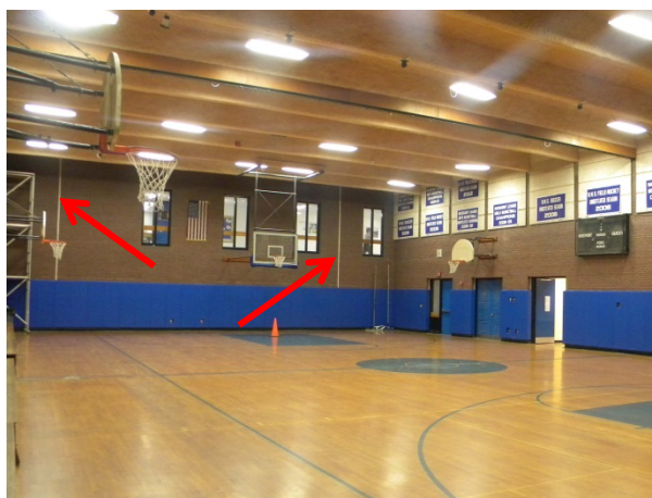
Figure C-24: Red arrows indicate the locations of expansion / control joints in the reinforced brick masonry wall at the gymnasium.
