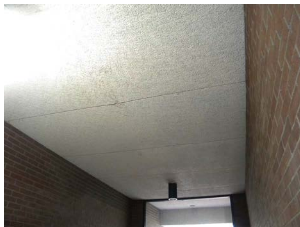
Figure C-13: Original Tectum form plank ceiling at typical stairway.
