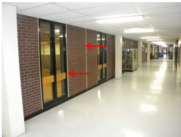
Figure C-27: Original interior caulk removed (and replaced) at expansion and control joints and at joints between steel frames and masonry.
