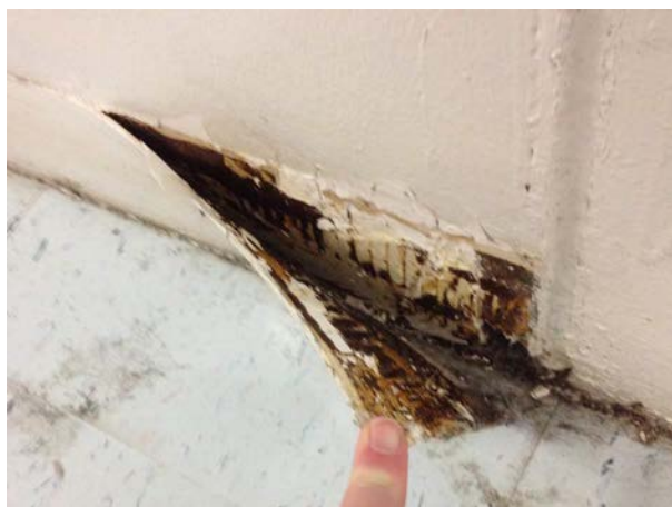
Figure D-07: Resilient base mastic.
