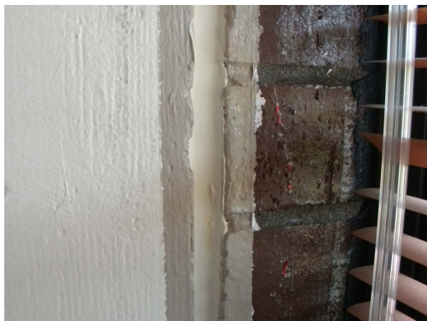
Figure C-26: Original interior caulk removed (and replaced) at joint between concrete column and brick pier.
