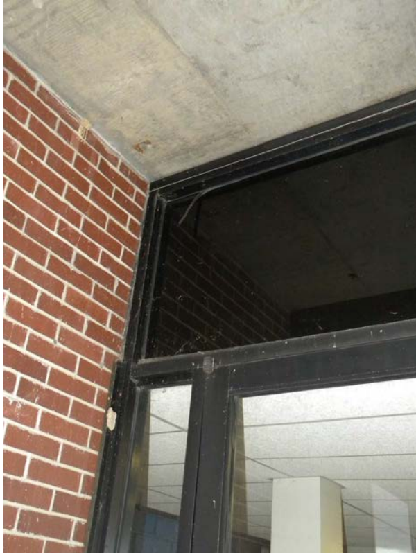
Figure H-09: Brick at jambs and concrete at head of one-story exterior door assembly.
