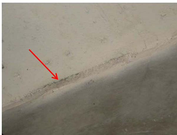
Figure G-32: Portion of Tectum form plank and mastic not fully removed during 2011 project.
