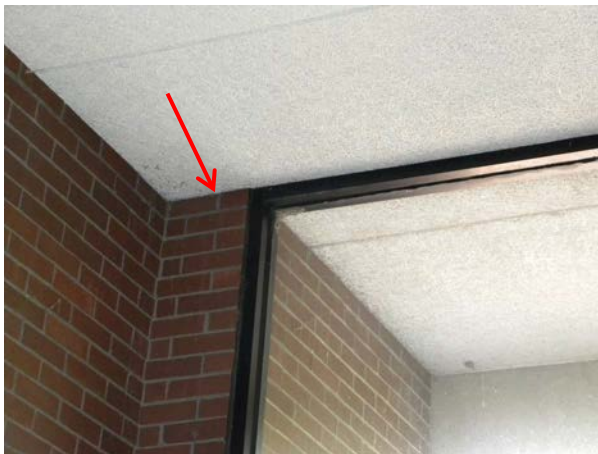
Figure G-09: Tectum form plank remaining at interior and exterior ceiling at stairways. Red arrow indicates 1'-0" step in brick veneer wall above which form plank extends.
