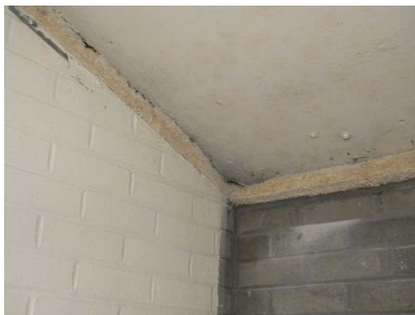
Figure G-21: Tectum form plank remaining at the tops of masonry partitions at the Band Room.
