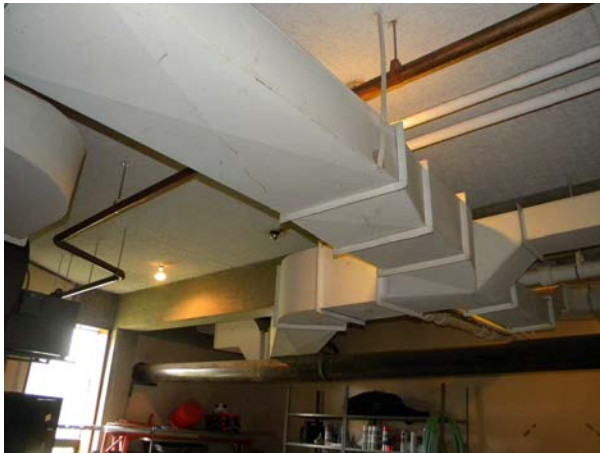
Figure G-18: Tectum form plank at Storage Room 153.
