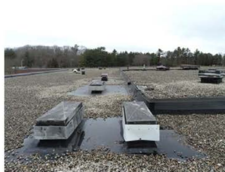
Roof Exhaust Fans
