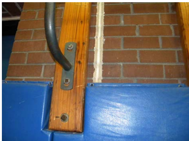
Figure G-34: Interior caulk at expansion / control joint in masonry wall is likely still in place behind wall pads in the gymnasium.
