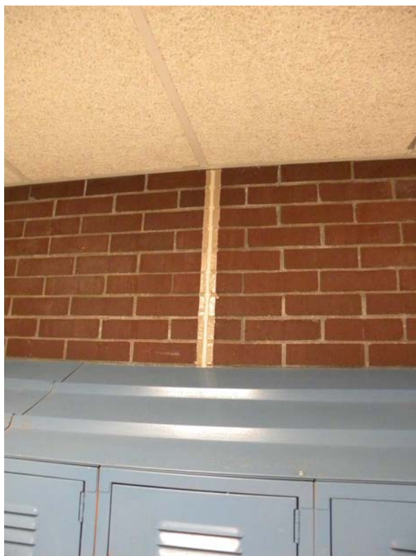
Figure G-33: Interior caulk at expansion / control joint in masonry wall is likely still in place behind the lockers.
