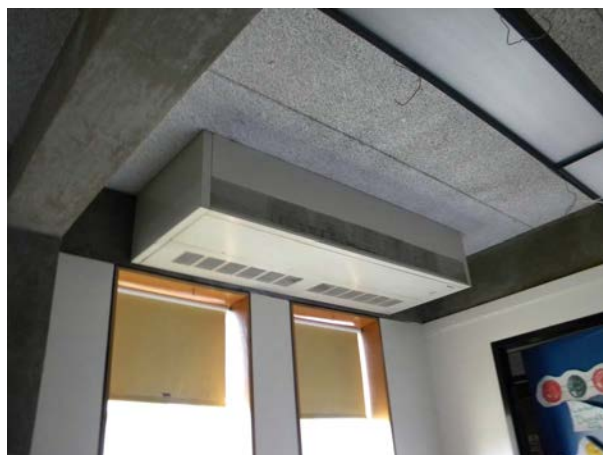
Figure I-10: Existing ceiling mounted unit ventilator. (Note: Photo is from before 2011 PCB Removal Project.)
