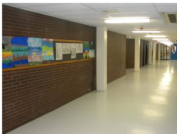
Figure H-29: Reinforced brick masonry walls at corridors.
