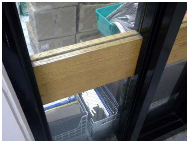
Figure D-11: Wood guard rail at fixed lite assembly.
