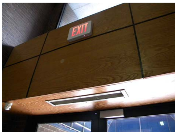
Figure H-10: Existing cabinet unit heater enclosure above typical two-story exterior door assembly head.
