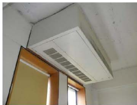
Ceiling Exposed Unit Ventilator
