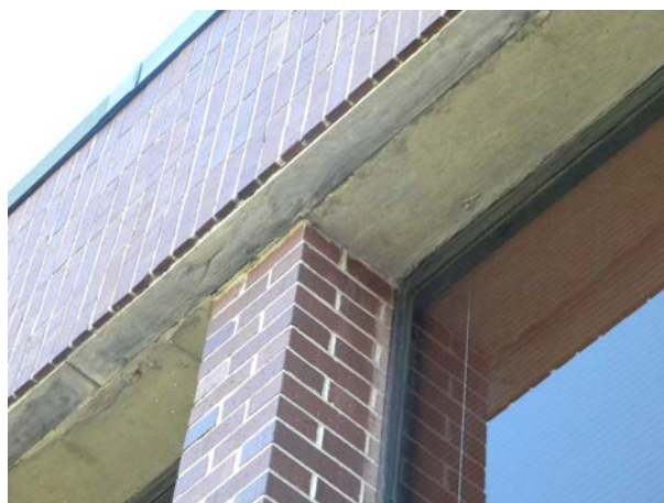
Figure D-01: Brick veneer at typical window jambs and cast-in-place concrete beams at typical window heads.
