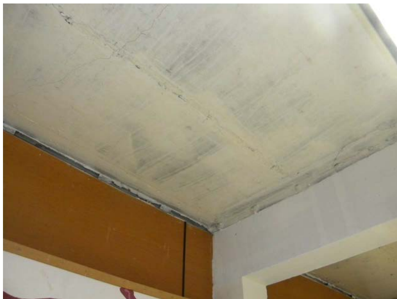
Figure C-18: Typical concrete slab, coated with bridging encapsulant, where Tectum form plank and associated mastics were removed.
