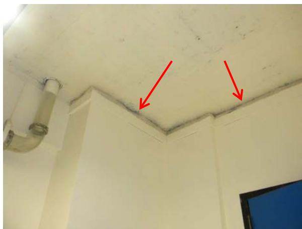
Figure C-20: Tectum form plank remaining at the tops of typical partitions.
