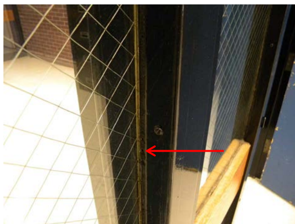
Figure D-04: Interior glazing compound at fixed lite sidelights and window walls.
