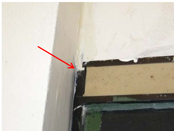
Figure G-37: Foam filler remains where concealed behind edge of existing chalk board.
