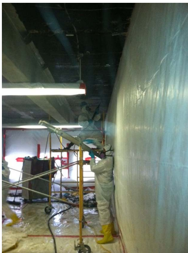
Figure C-16: Removal of existing Tectum form plank and associated PCB-containing mastic. [Photo courtesy of EnviroScience]
