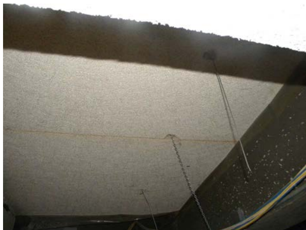
Figure G-31: Tectum form plank concealed above suspended ceiling at corridor.
