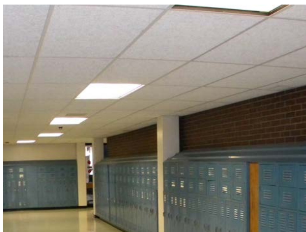
Figure D-06: Tectum acoustical ceiling panels at typical corridor.
