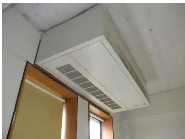
Figure C-21: Tectum form plank remaining above typical ceiling-mounted unit ventilators.
