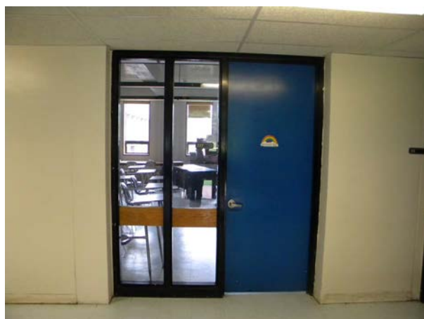
Figure H-31: Steel-framed door and fixed lite assembly from corridor to classroom.
