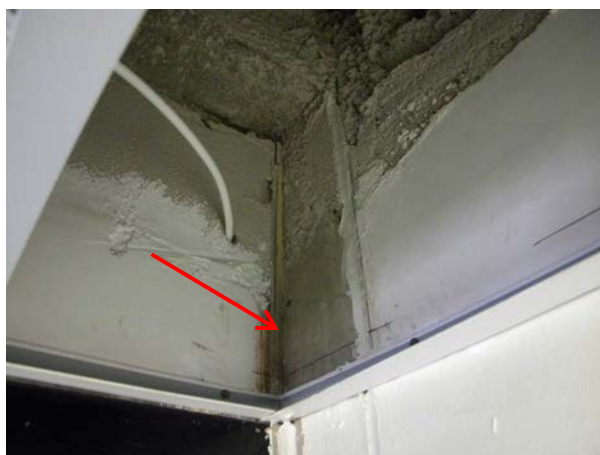
Figure G-39: Red arrow points to segment of foam filler between metal corner bead and concrete column that was not removed in 2011 from above the suspended ceiling at this location.
