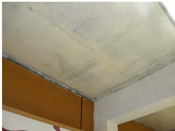
Figure H-25: Cast-in-place concrete columns, beams, and slabs.
