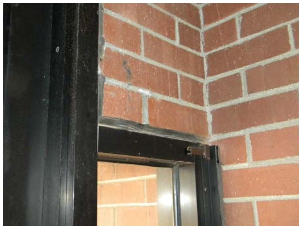
Figure C-07: Interior caulk at perimeter of door frame. (Note: photo is from before 2011 removal project.)
