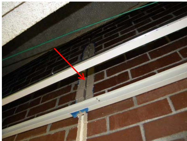
Figure G-35: Interior caulk at expansion joint removed above suspended ceiling tiles.
