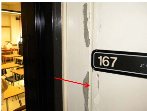
Figure H-24: Joint at concrete column to plaster wall.
