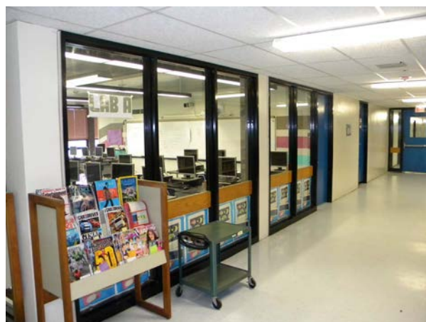
Figure H-32: Steel-framed door and fixed lite assemblies at Media Center.
