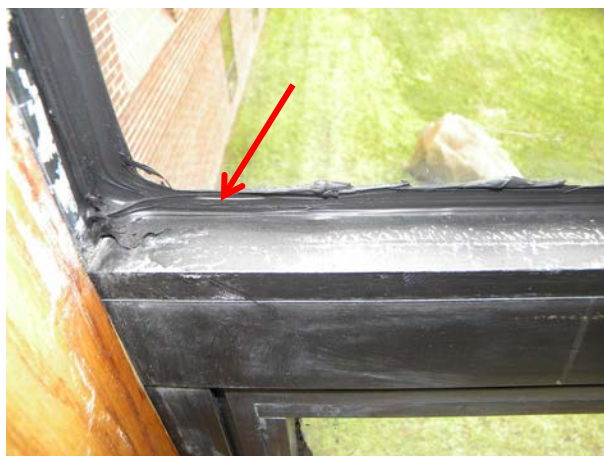
Figure C-11: Sealant applied over interior glazing compound at typical windows as part of the 2011 removal project.
