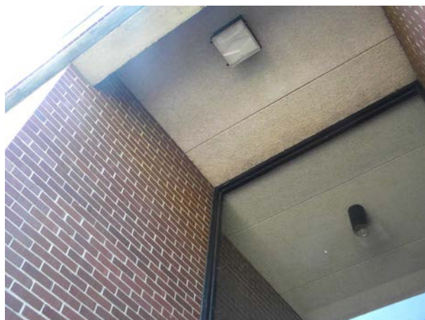
Figure C-19: Tectum form plank remaining at exterior and interior stairway / entrance ceilings.
