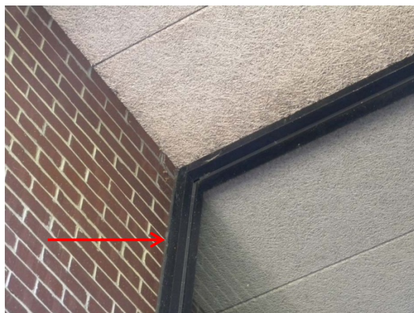
Figure G-01: Exterior PCB-containing caulk at door assemblies above 8'-0".
