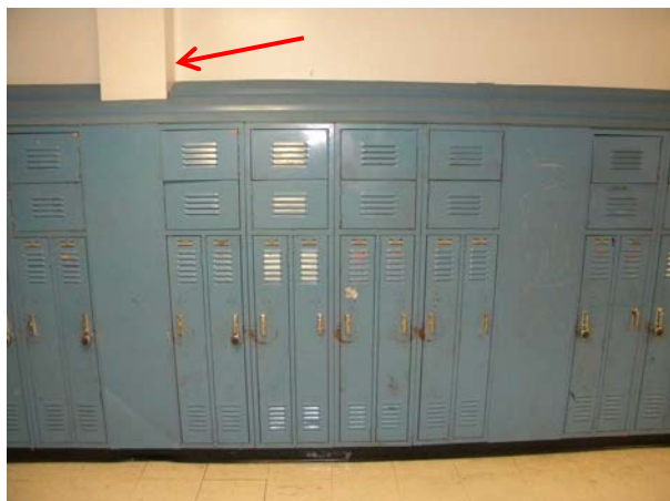
Figure G-36: Interior foam filler at joints between concrete columns / beams and steel stud / plaster partitions is indicated by red arrow. This joint with foam filler likely extends down and remains behind existing lockers.
