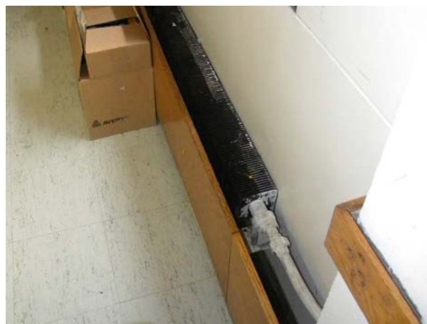
Figure I-11: Existing finned tube radiation at perimeter walls.
