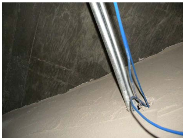
Figure D-05: Bare concrete slab without Tectum form plank above suspended ceiling areas.
