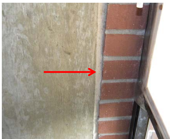
Figure C-23: Interior caulk at joint between cast-in-place concrete and brick.
