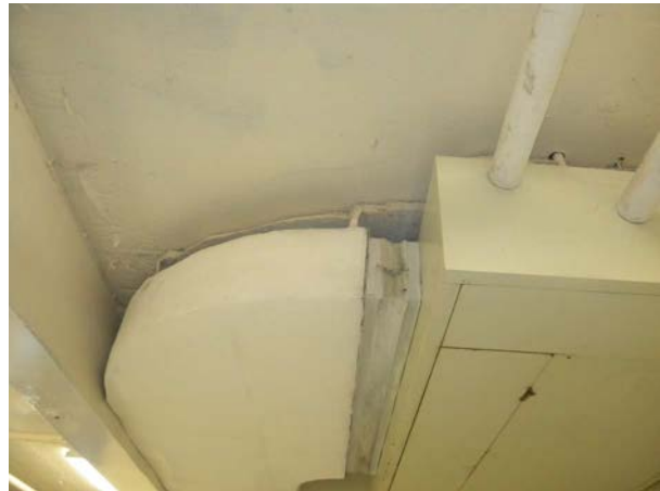
Figure G-25: Tectum form plank above mechanical equipment and ductwork in Special Education Room 155.
