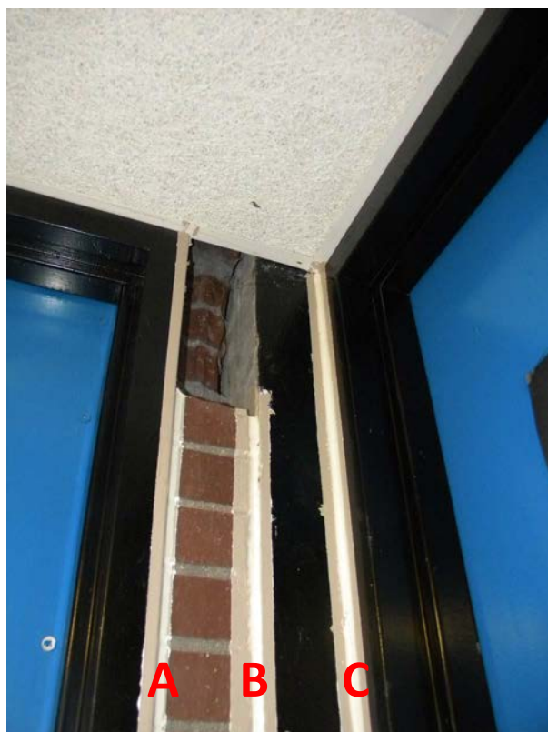
Figure C-25: Interior caulk joints at steel door frames to brick (A), brick to concrete (B), and concrete to steel door frames (C). (Note: this is a post-remediation photo.)
