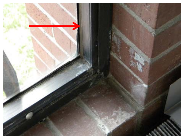
Figure C-10: Interior glazing compound at typical windows.
