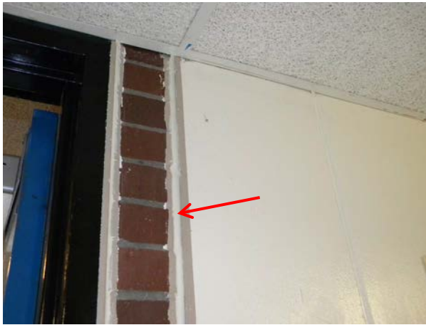
Figure H-16: Joint at brick to concrete at stairways. (Note stripes of gray epoxy encapsulant at either side of existing joint applied in 2011.)
