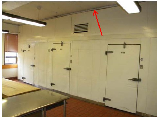
Figure G-17: Tectum form plank above built-in refrigerators and freezers.
