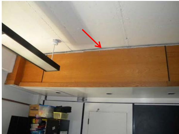
Figure G-26: Typical soffit construction above movable partitions.
