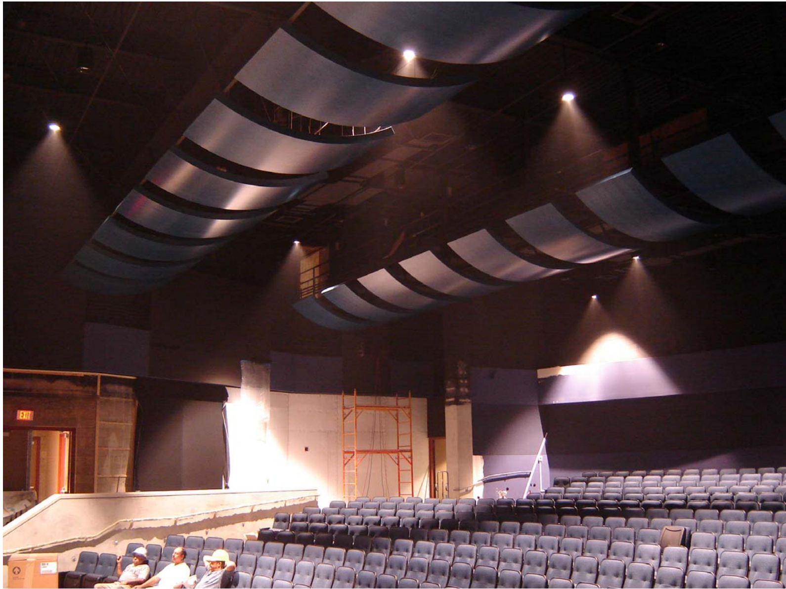
West Ranch High School Theater – Curved Wooden Ceiling Panels
