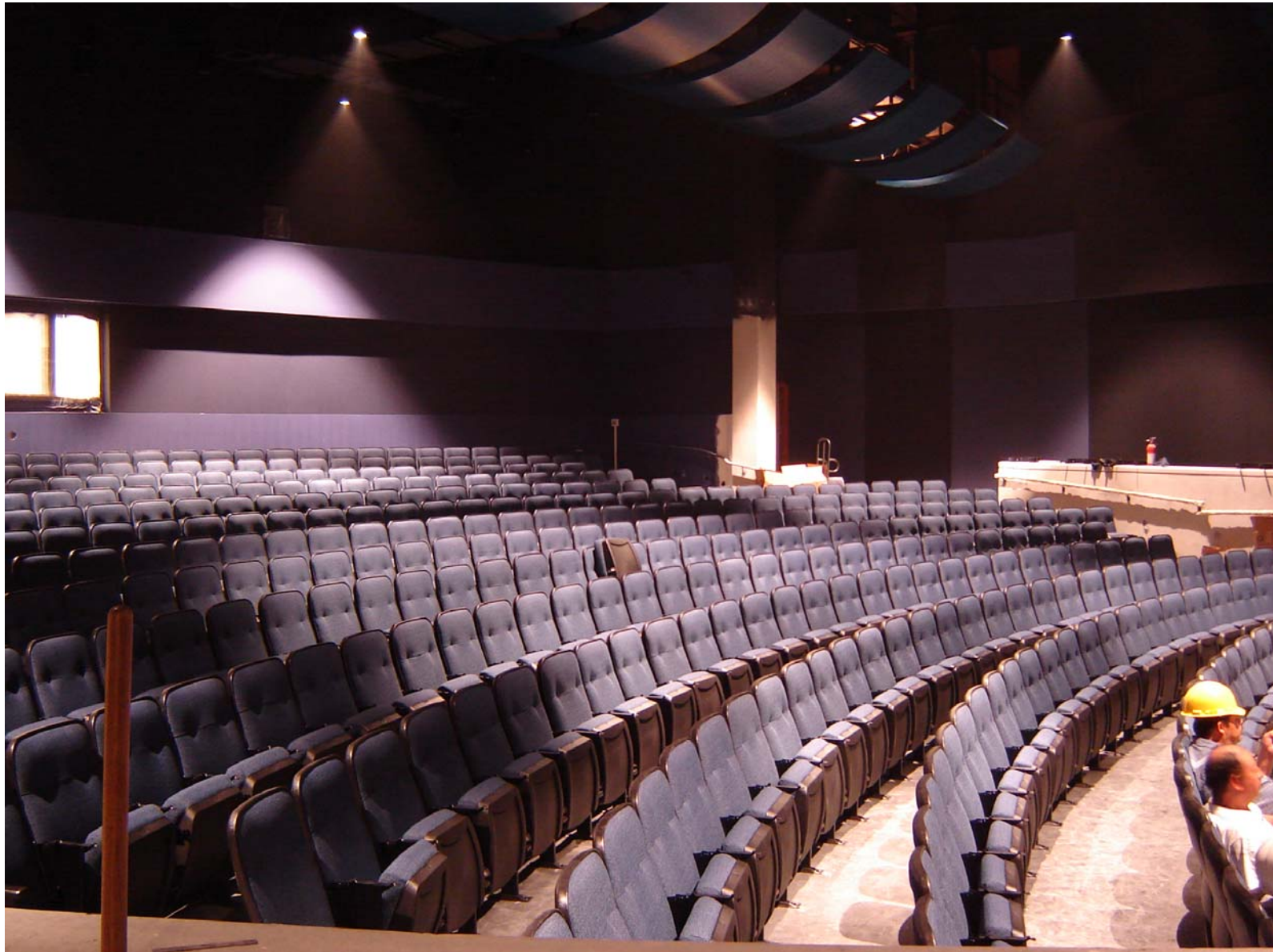
West Ranch High School Theater – Seating Installation Underway
